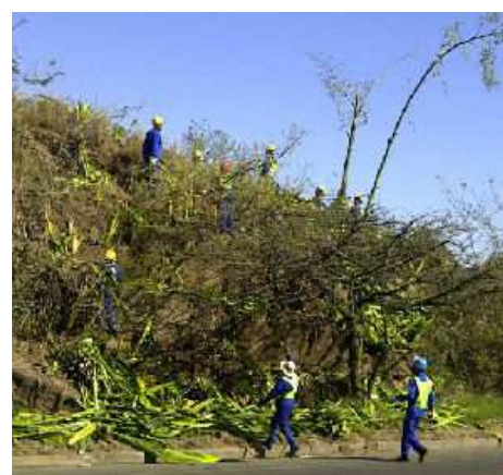
During clearing operations
